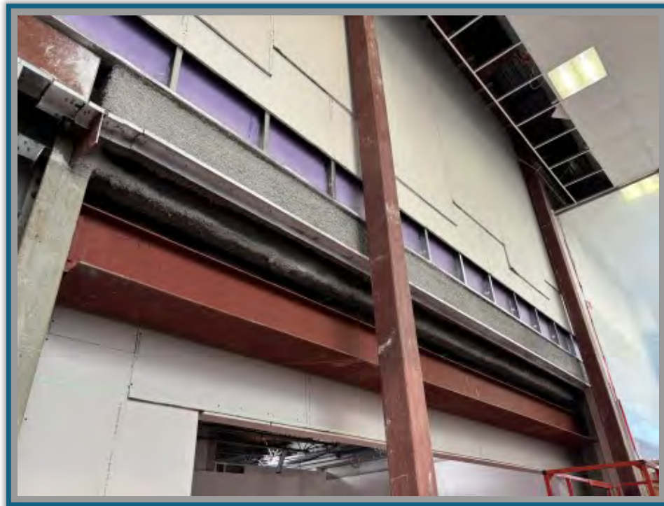
Upper Lobby walls (above new opening for north hallway) being replaced after steel installed.
