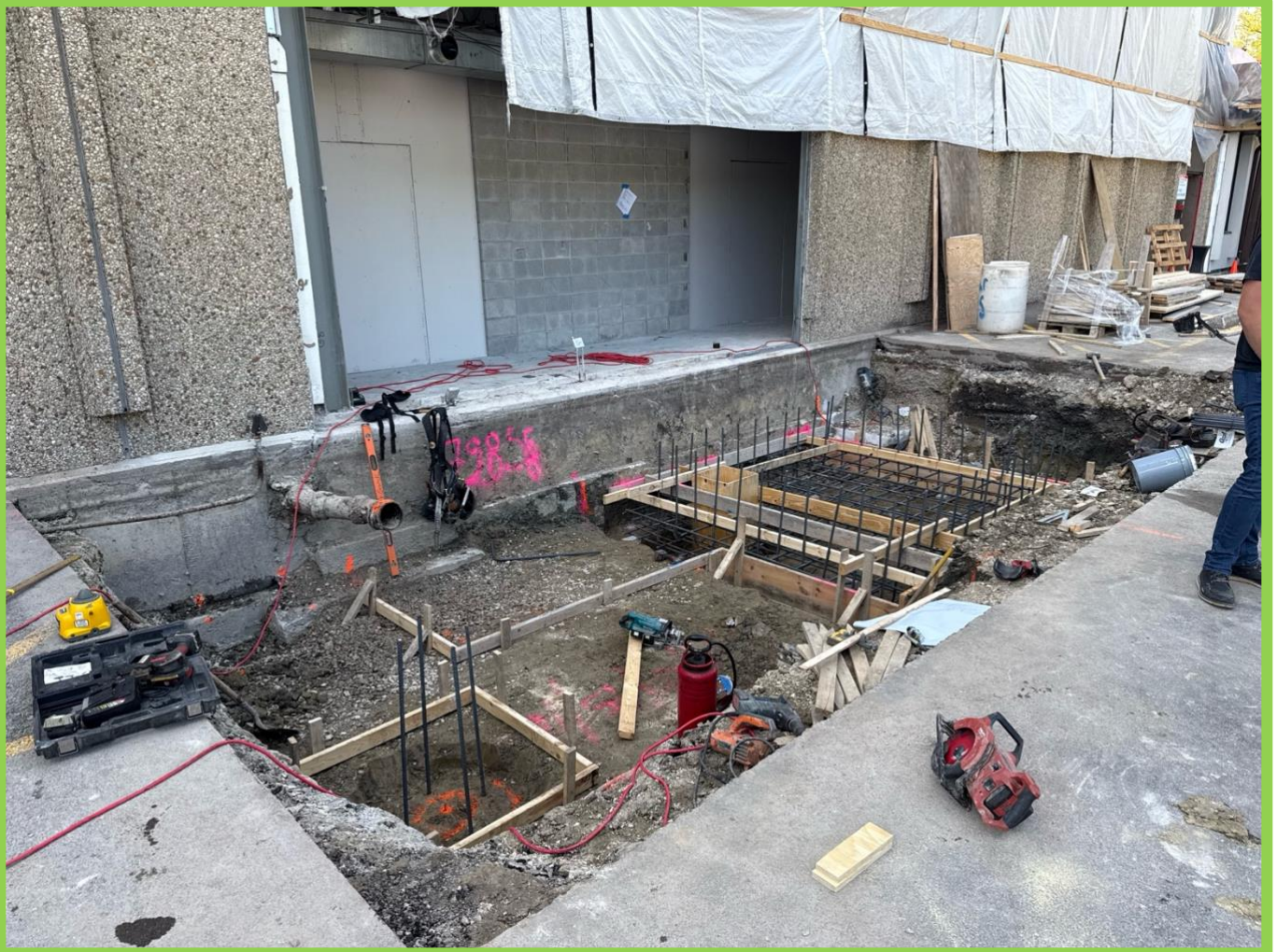
Pit for elevator ready for foundation. Opening in building with new North Entry on left, elevator on right,
